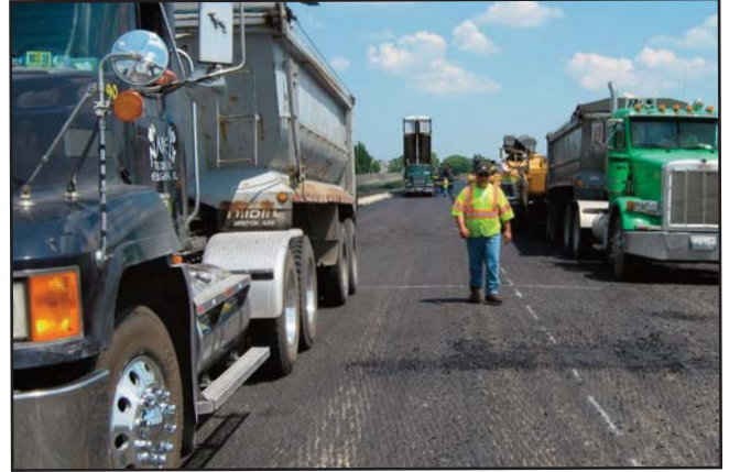
An ITCP should provide rules for workers if they must pass vehicle paths (Source: ARTBA).
