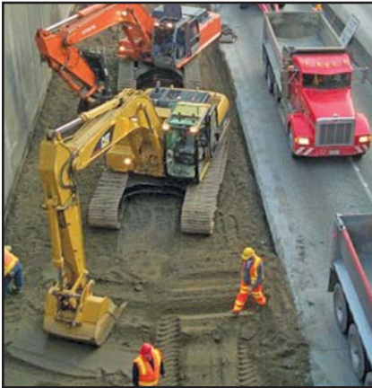
An internal traffic conflict between workers on foot and equipment (Source: pavementinteractive.org ).
